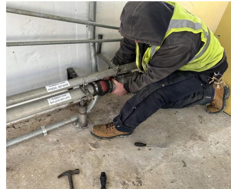
RWSA staff repairing the air line coupling
